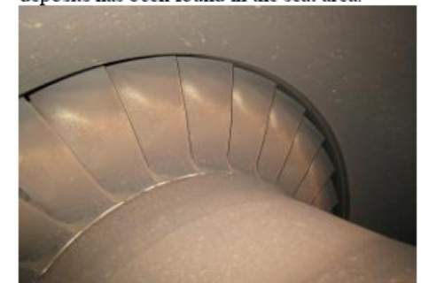
Inspection area #9: The turbine blades were found without major deposits.
